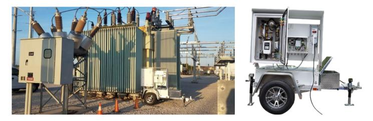
IP&L used Vaisala's Optimus<sup>™</sup> Mobile multi-gas DGA Monitor, the OPT100 Mobile and Delta-X Research's Transformer Oil Analyst<sup>™</sup> software with Monitor Watch<sup>™</sup> to detect and identify faults on a suspect transformer. This was done without taking the transformer offline by using a mobile DGA online monitor and feeding its information to a cloud-based analytic software tool.
